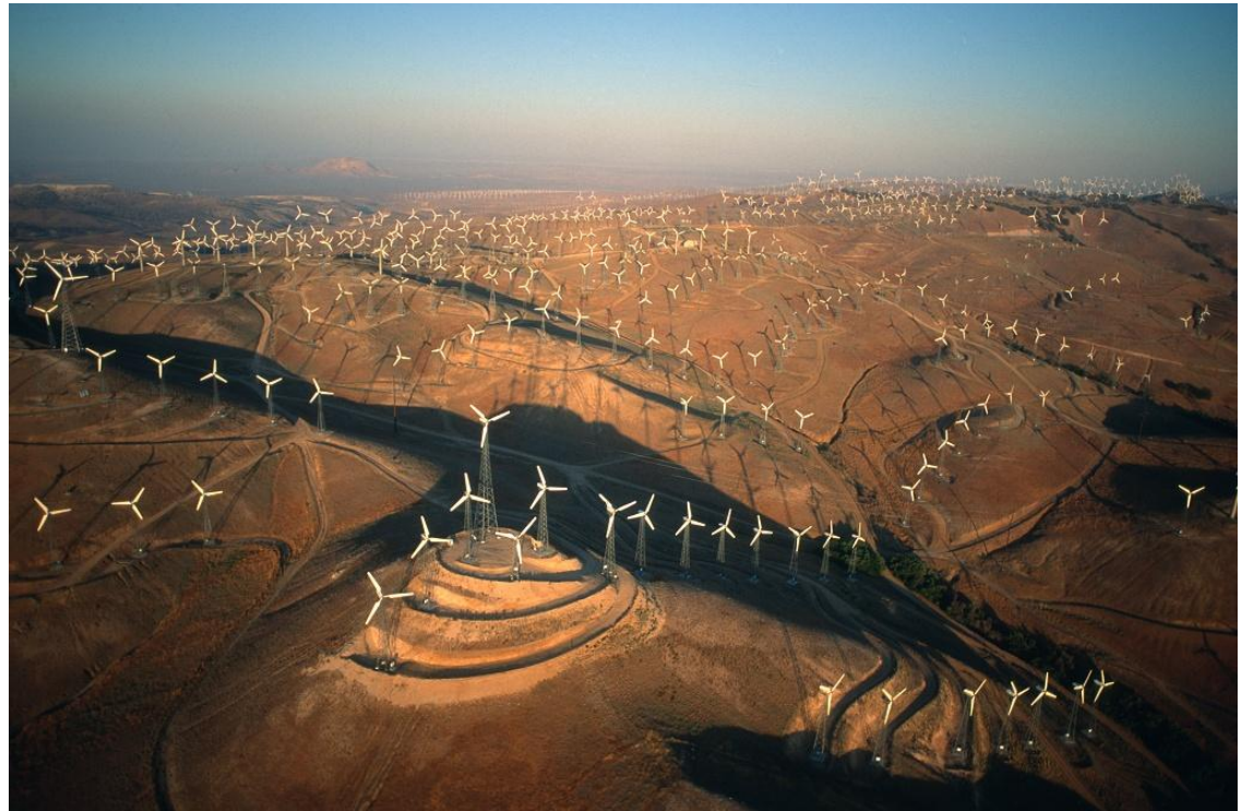
Tehachapi Wind Farm (California - USA)
